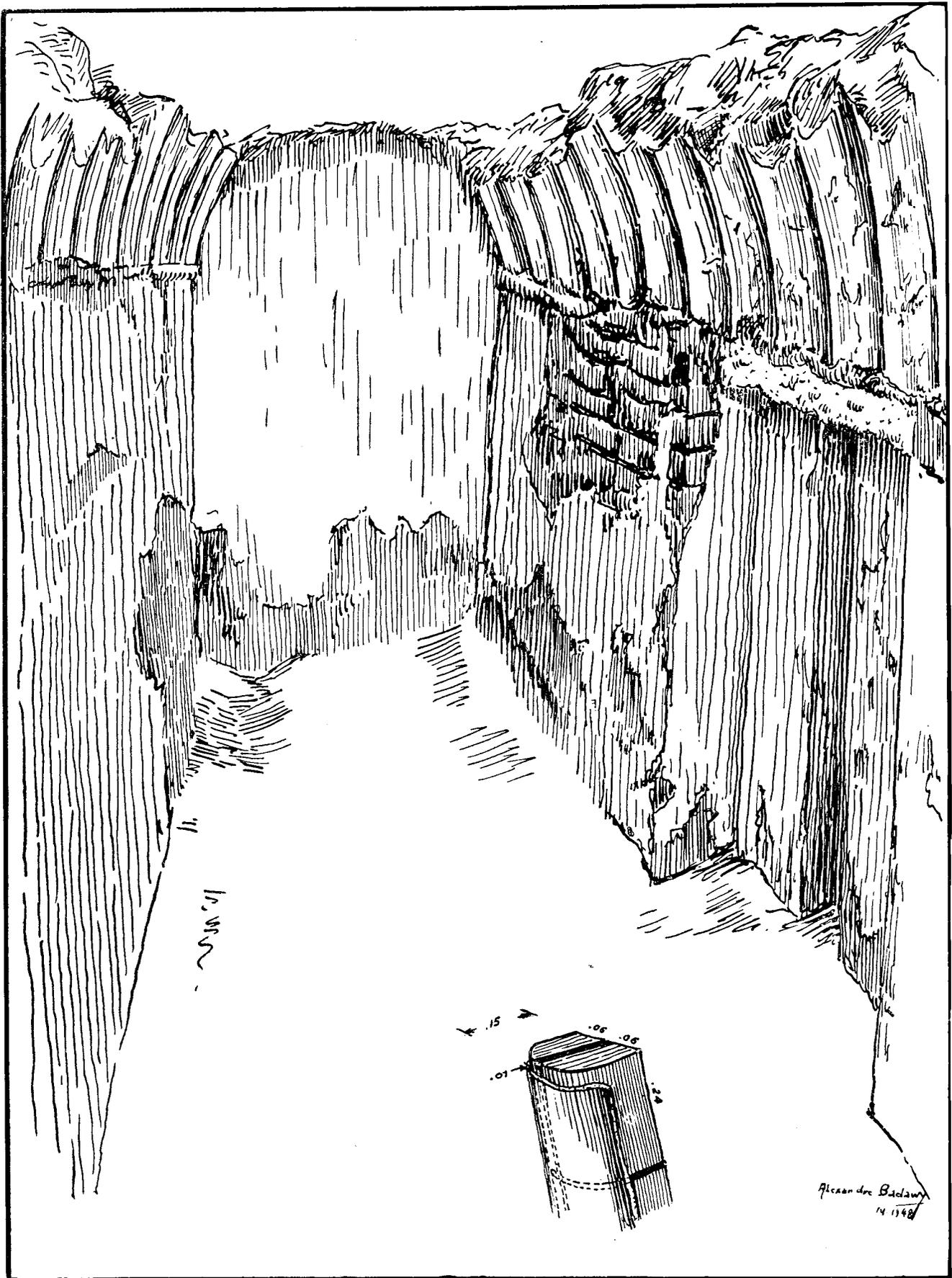
FIG. 110.—Ribbed catenary vault at Giza
